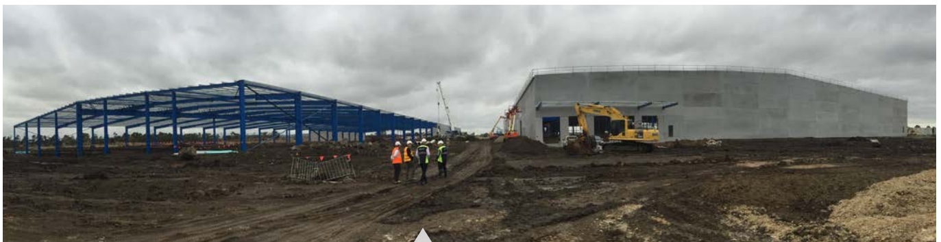
Inspecting the progress at the new Epping Site
