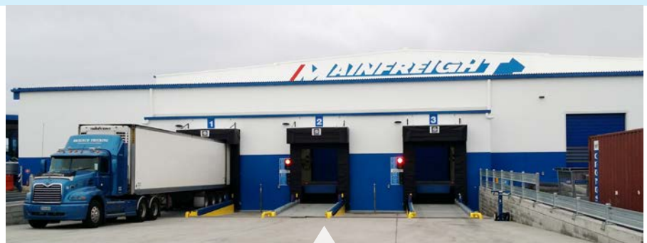
New Westney Road Warehouse – Loading Docks
