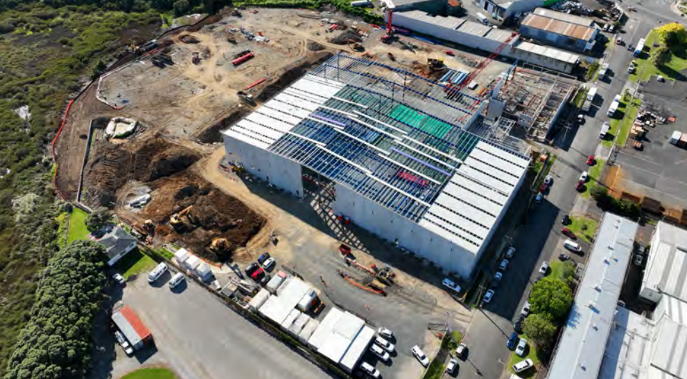
Beach Road construction
