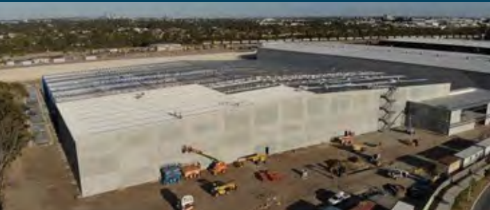
22 December 2022 – Structure going up
