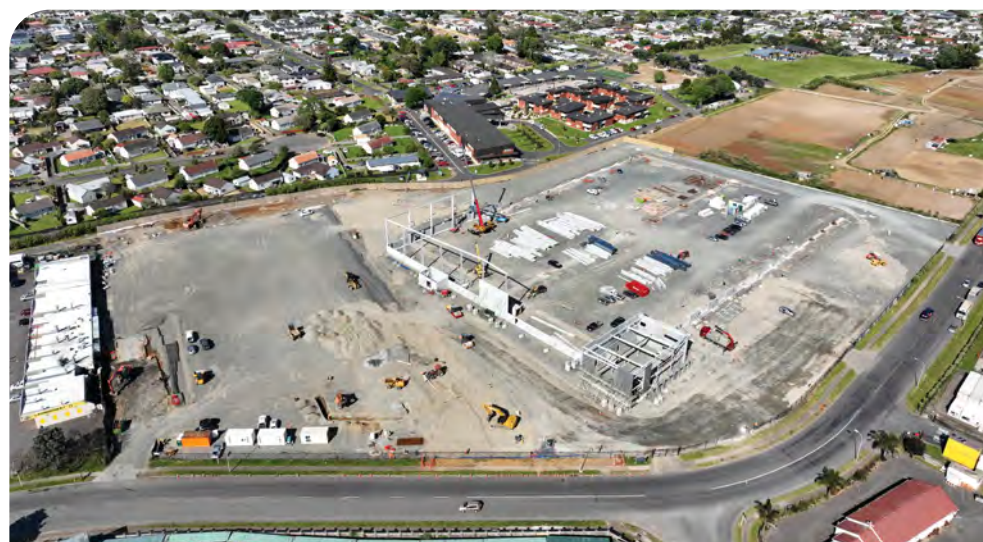
Savill South construction
