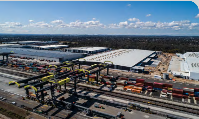
Moorebank Intermodal Precinct
